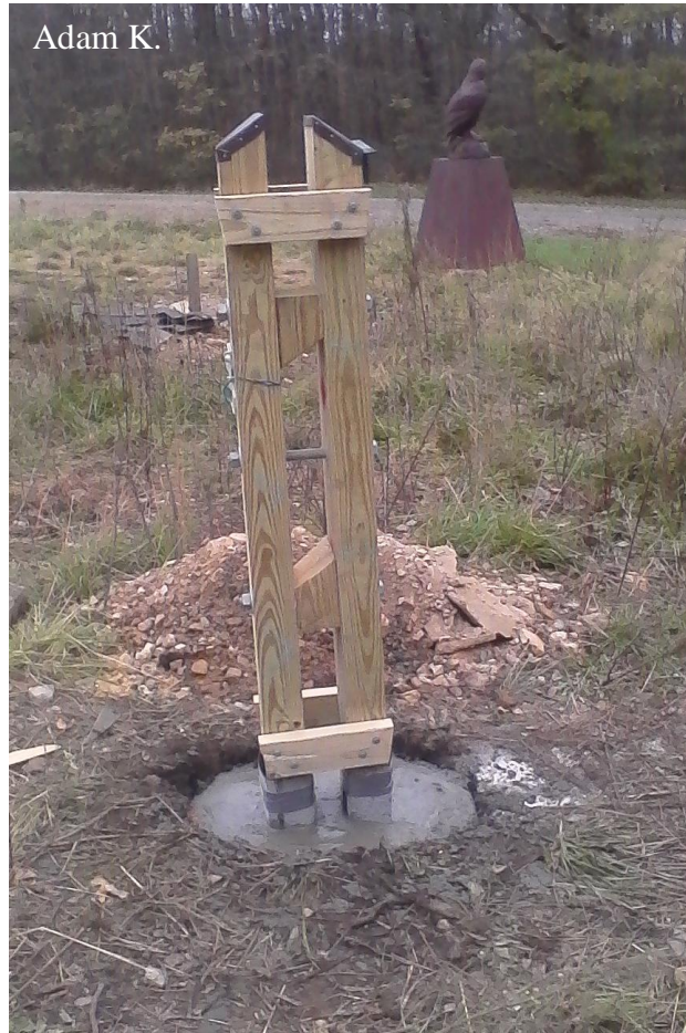
Above: The foundation for the bat box that will be a permanent fixture at the Allegheny Front Hawk Watch.
